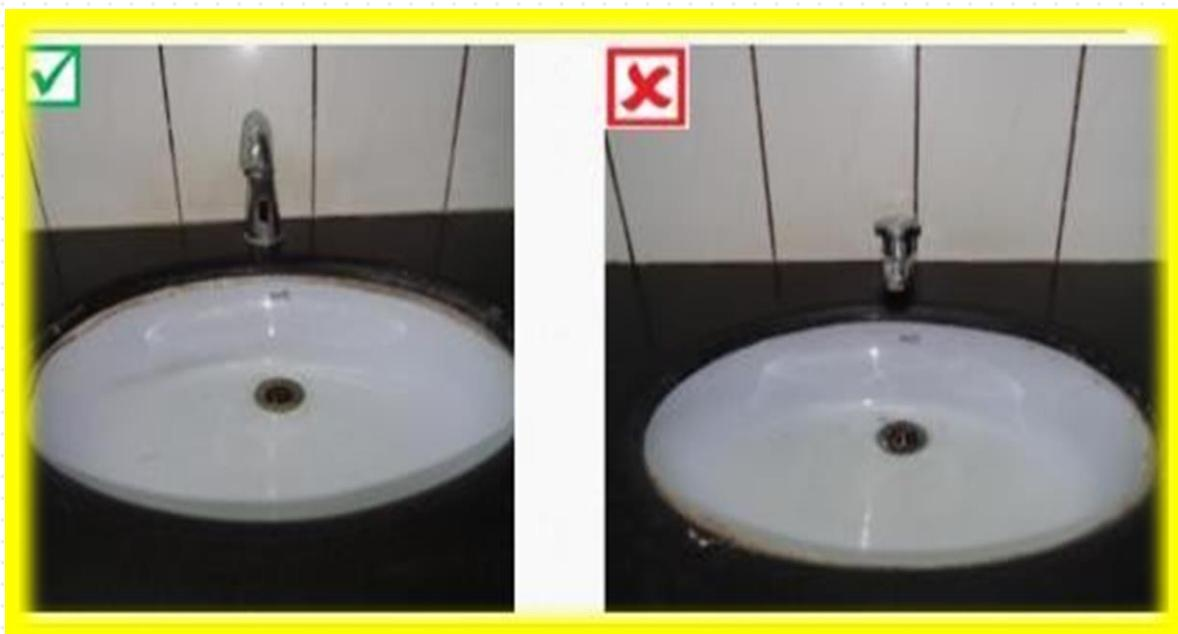
**Fig: Touch free (hands free) tap sat wash basins to avoid cross contamination**
